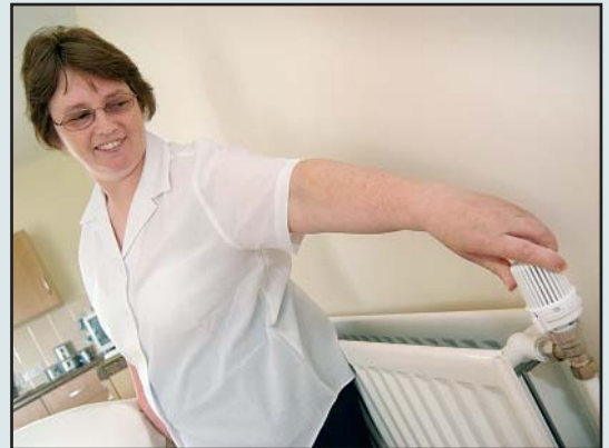
Thermostatic valves on radiators can help to make substantial energy savings.
