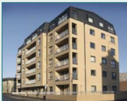
670 Argyle Street provides 24 flats for wheelchair users in the heart of Glasgow.
